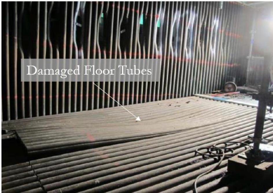
**Fig. 2 - Deposits impacting the boiler floor can have serious consequences on the floor tubes**
